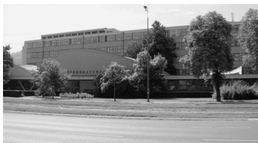
SLIKA 13. Zgrada Instituta za hemiju i fiziku godine 2014. FIGURE 13. The building of the Institute of Chemistry and Physics in 2014
